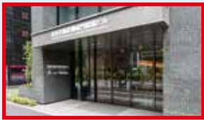
Arrive at Bellesalle Onarimon Ekimae (The entrance of SUMITOMO FUDOSAN ONARIMON EKIMAE BLDG.)
